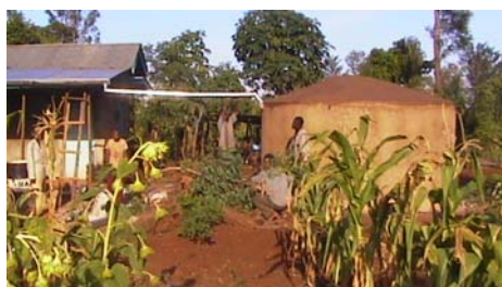
Completed rainwater harvest tank
