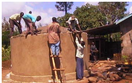
Construction of rainwater harvest tank in Rombo
