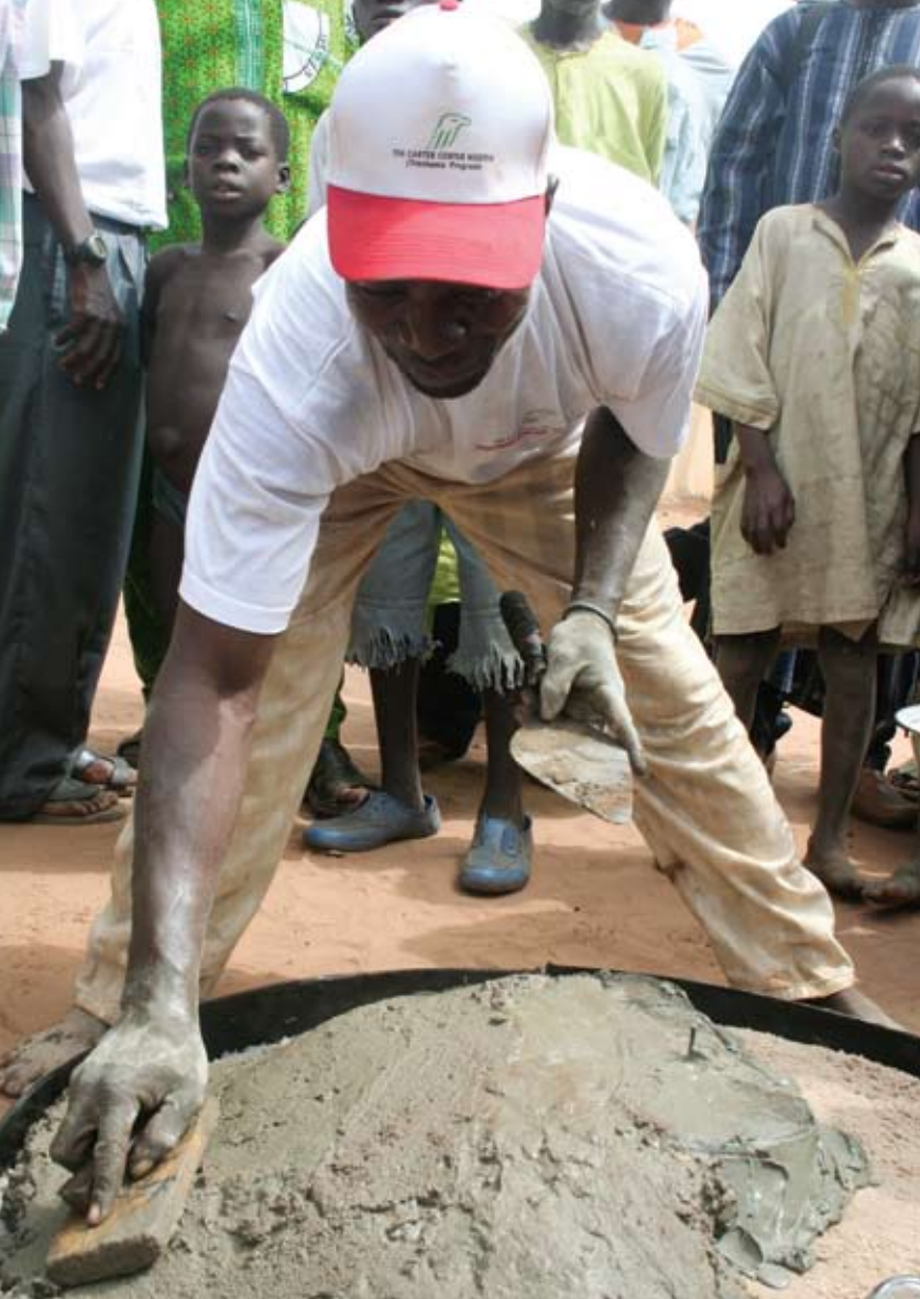
A mason builds a latrine slab in Nigeria.
